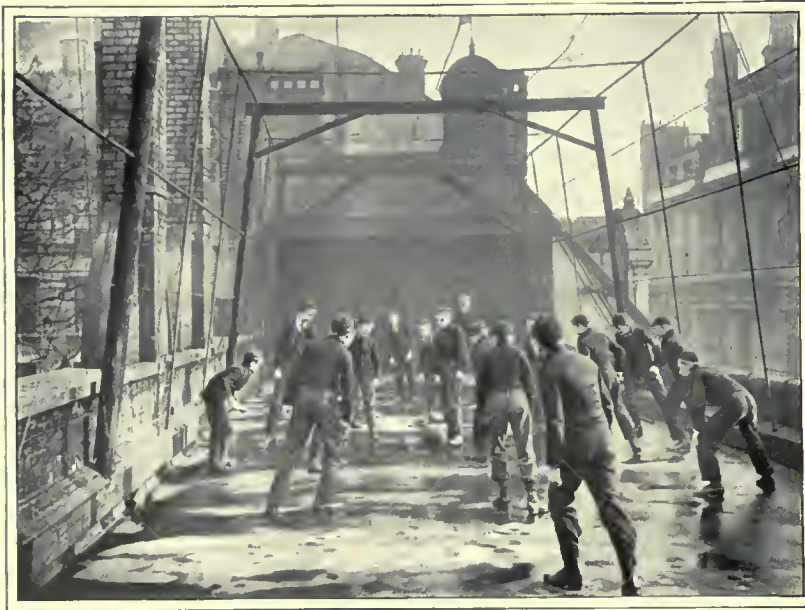
ON THE ROOF OF ST. PAUL'S CATHEDRAL CHOIR SCHOOL.
